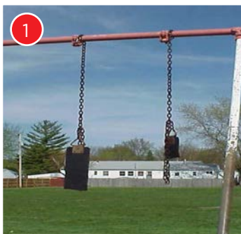
1 Swing chain should be unwrapped/inspected and broken swing seat should be replaced.
