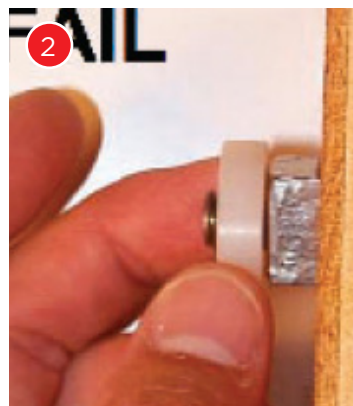
2 This bolt end is an unsafe protrusion.
