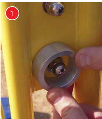
1 Gauges are used to test the compliance of all projections. This projection is in compliance because it does not extend beyond the face of the gauge.
