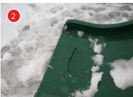
This tear could be an entanglement hazard.
